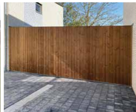
Thermowood verticale beplanking
