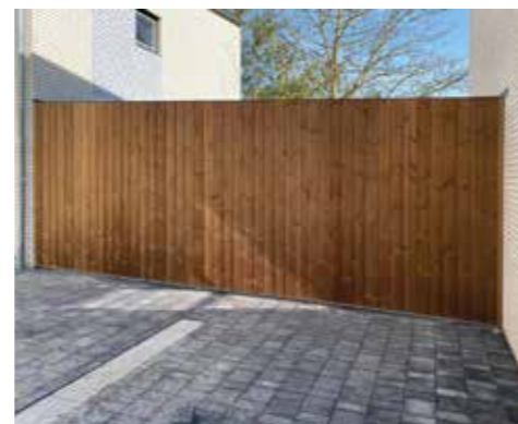
Thermowood verticale beplanking
